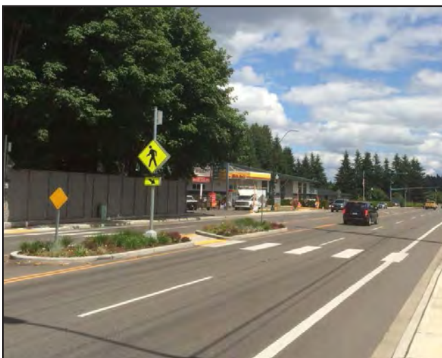
DIAGONAL MID-BLOCK CROSSING COURTESY WSDOT DESIGN MANUAL
